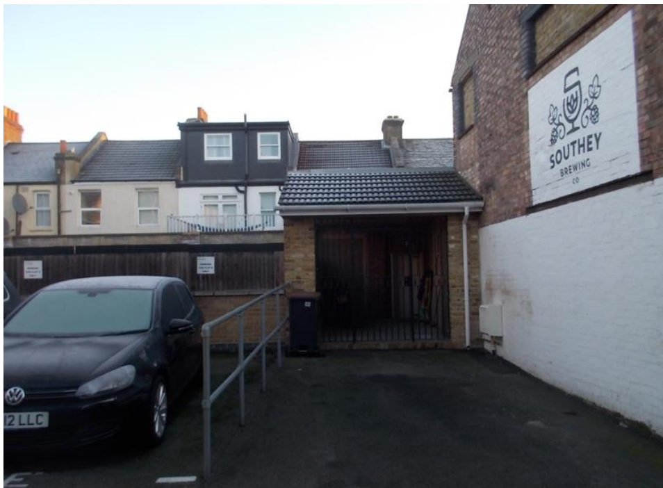
Figure 3 Existing entrance to building
